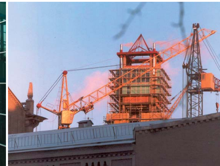
Construction in the capital In a new office center
